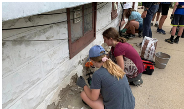
Volunteers patch cement on the foundation of a home during Hands of Hope in Milwaukee.
